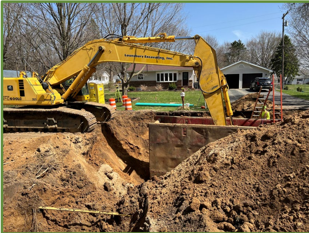
Sanitary and Storm Installation
