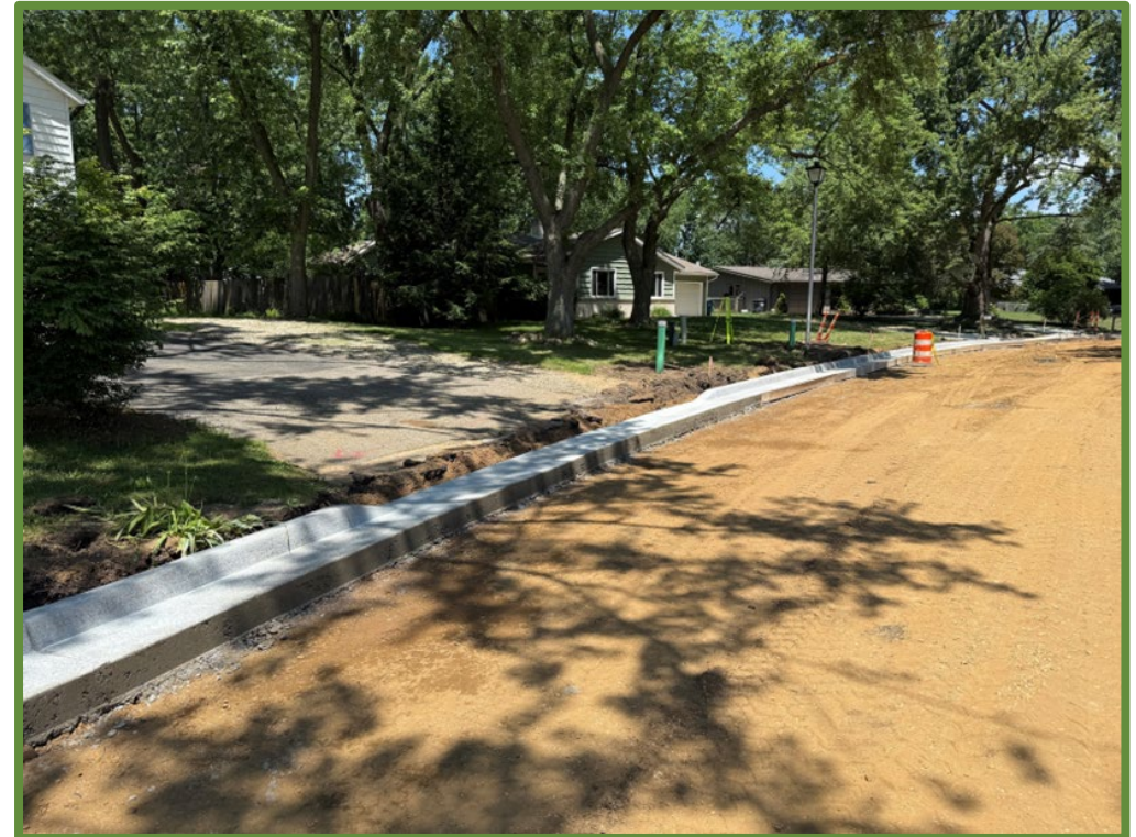
Curb and Gutter Replacement
