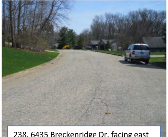
238. 6435 Breckenridge Dr. facing east
