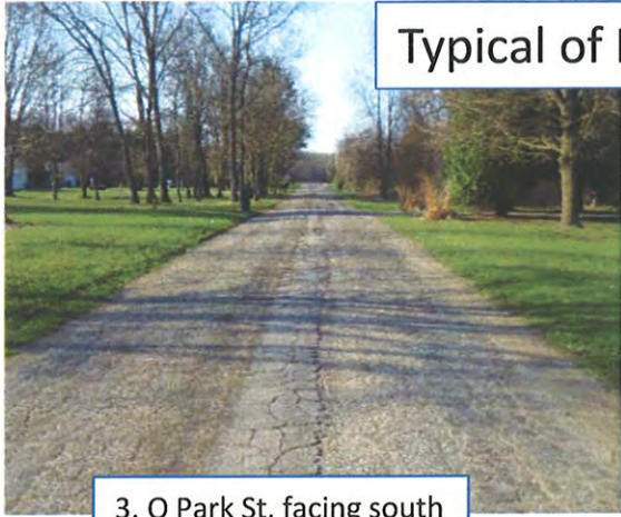
3. O Park St. facing south
