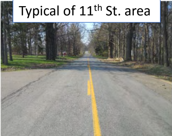
20. S. 11 th St at driveway to Kal. Christian facing south
