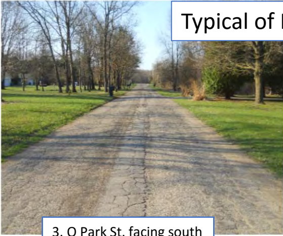
3. O Park St. facing south
