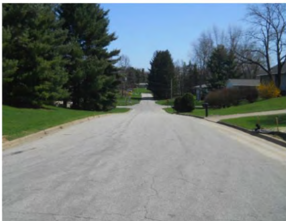
158. Valley View Dr. at E. Ridge Cir. facing east
