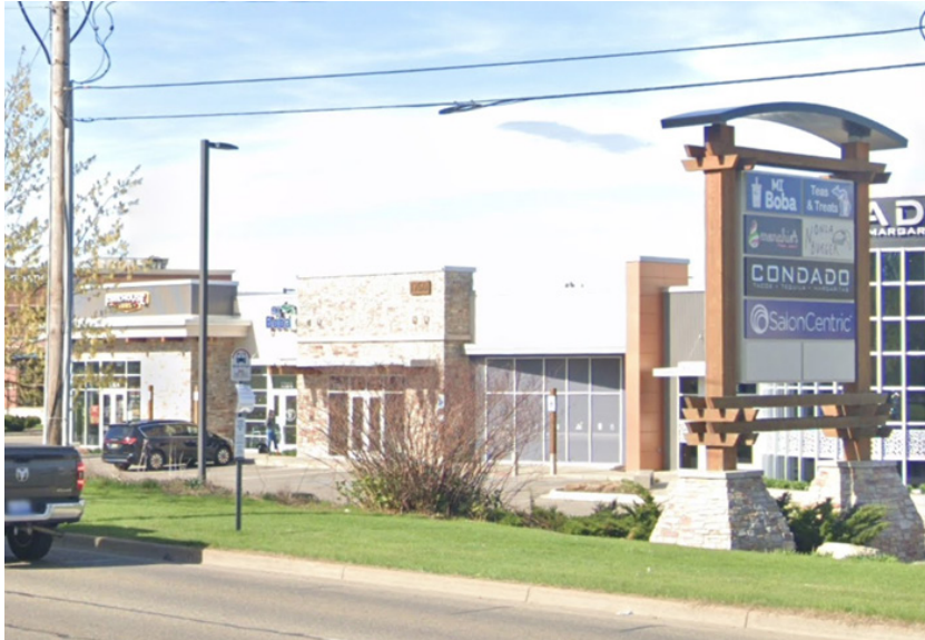
Transit stop on grass, no concrete pad and sidewalk connection to make the stop wheelchair accessible.
