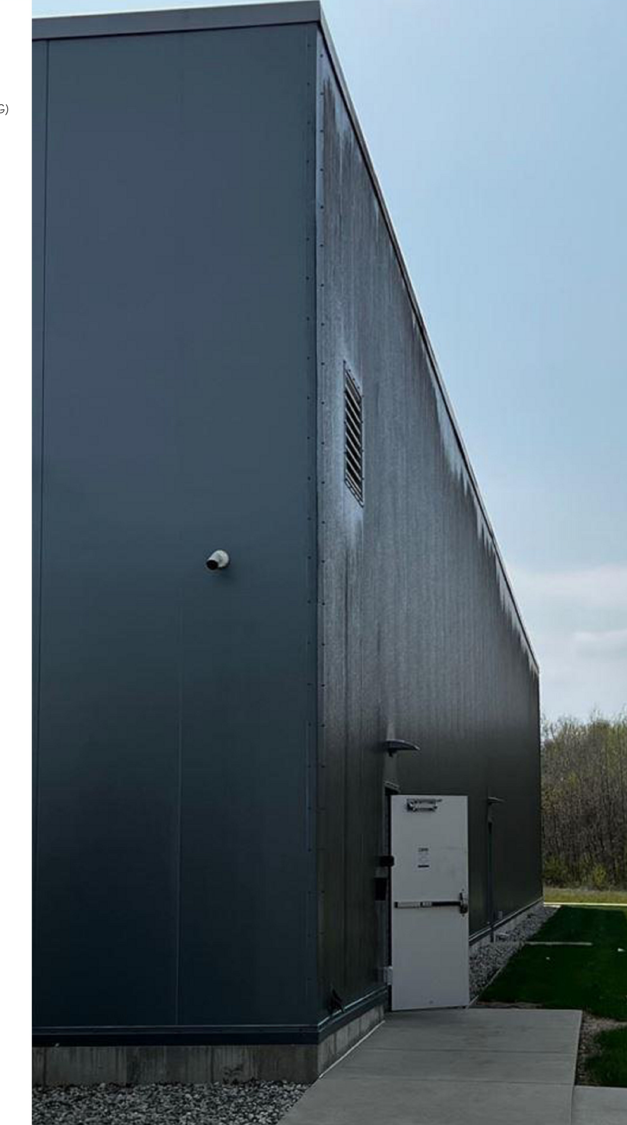
EXISTING EXTERIOR METAL PANELS (NEW FACILITY EXPANSION TO MATCH)
