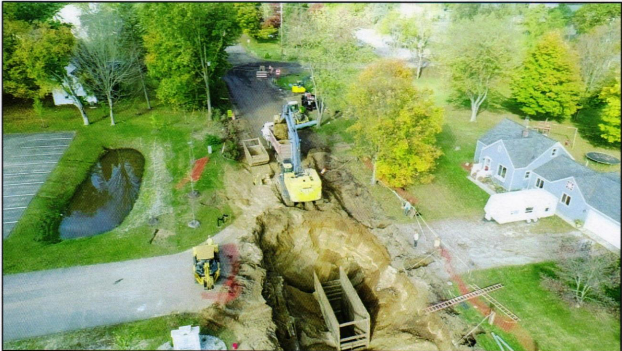
A drone's view of the 30-ft sewer trench in KL Avenue.
