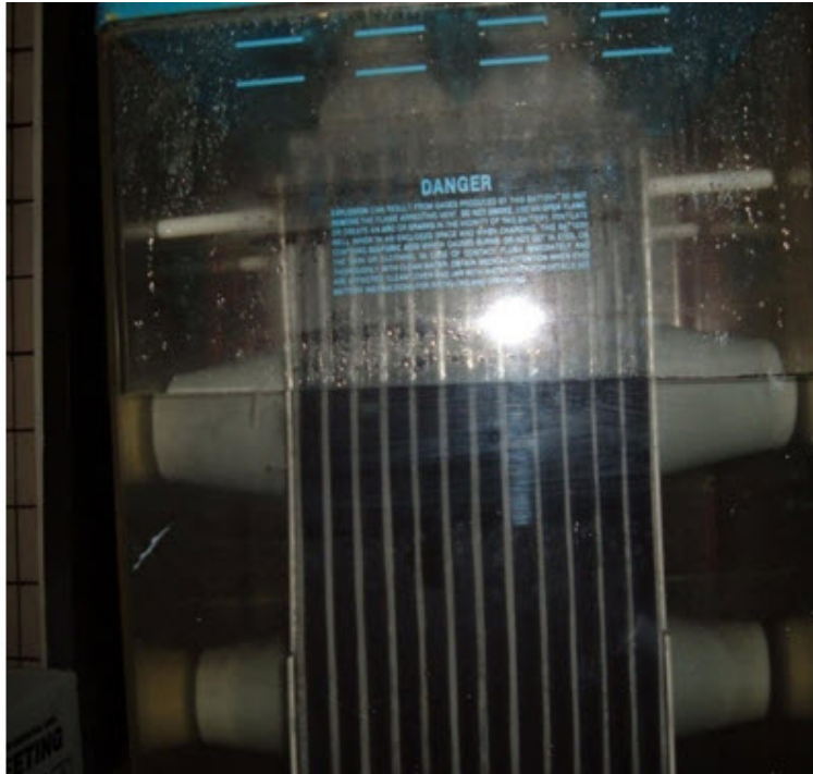
Fig. 3.3.3.4. Severely low electrolyte observed at visual inspection
